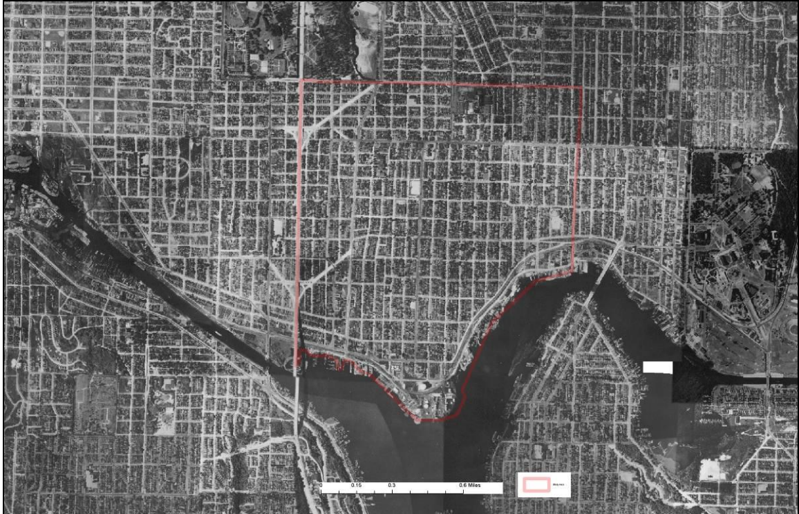
Figure 2--Aerial Photo Showing Recently Constructed Highway 99, 1936
